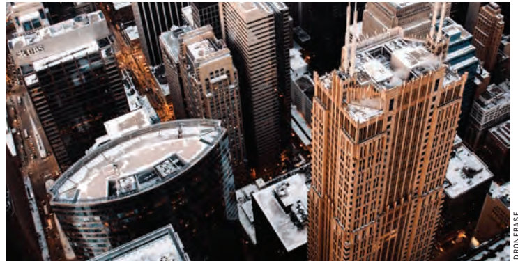
The use of drones is ideal for inspecting rooftop and HVAC conditions on high-rise buildings in dense cities.
