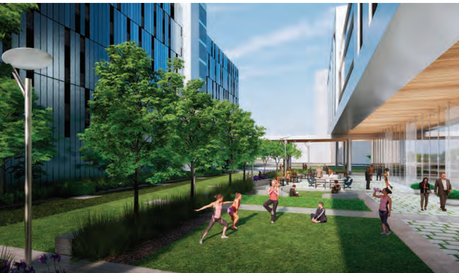
The plan for the Christus Health headquarters in Irving, Texas, incorporates outdoor spaces to provide greater safety and to allow for exercise and recreation.
